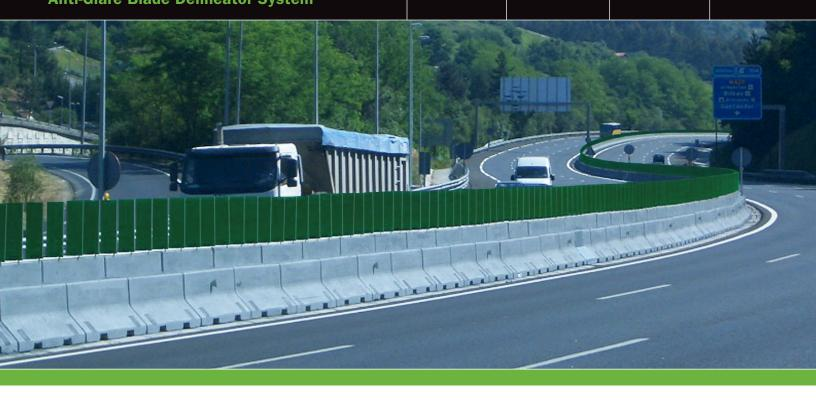
The Safe-Hit<sup>®</sup> Glarescreen is a vertical blade delineator system that is used to delineate both temporary and permanent medians and block out headlight glare of oncoming traffic.
